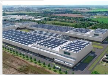
Award of precast solutions for the battery gigafactory in Sagunto.
