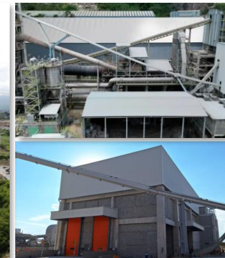
New alternative fuels facilities in Mexico and Colombia
