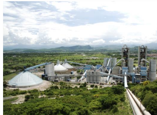
Capacity increase at the Tepetzingo plant (Mexico)
